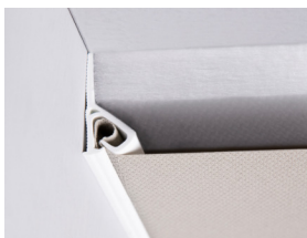
Clipso ceiling installation with PCW profile.
