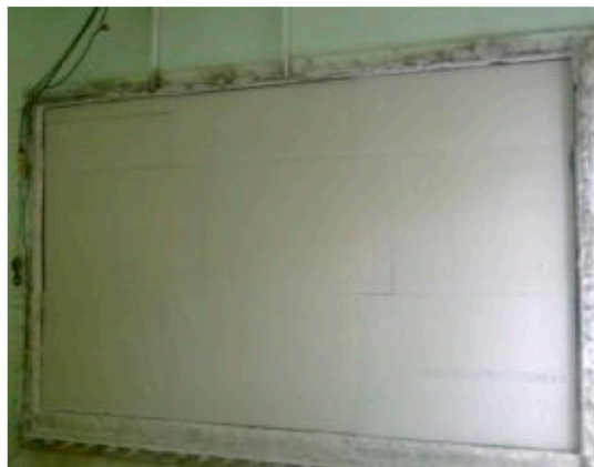
Finished wall with 12.5 mm GKB gypsum board
