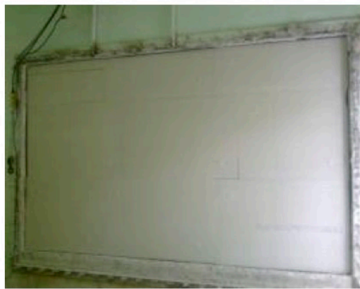
Finished wall with 12.5 mm GKB gypsum board
